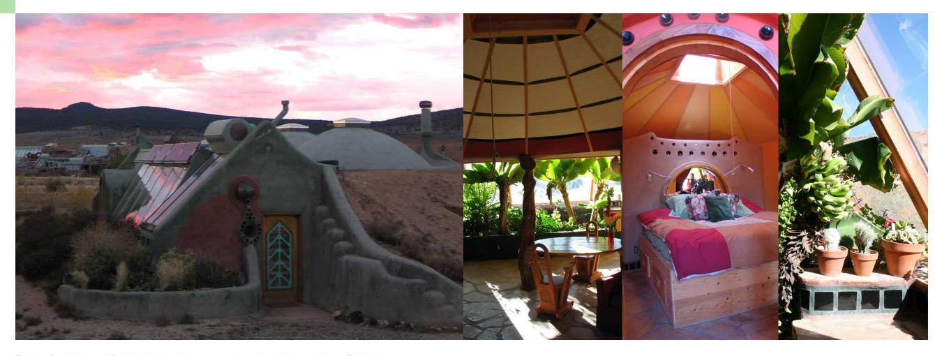
The Hut Earthship is two Earthship Hut Modules connected by a sloped face greenhouse. This design evolved after a hurricane-relief project in Honduras. The Huts are built with circular shaped rooms built with tire walls. The domed roof structures are built on the ground with steel rebar bent, wired together, sheathed in wire mesh and lifted in place on top of the tire walls. The roof is then plastered with cement.
