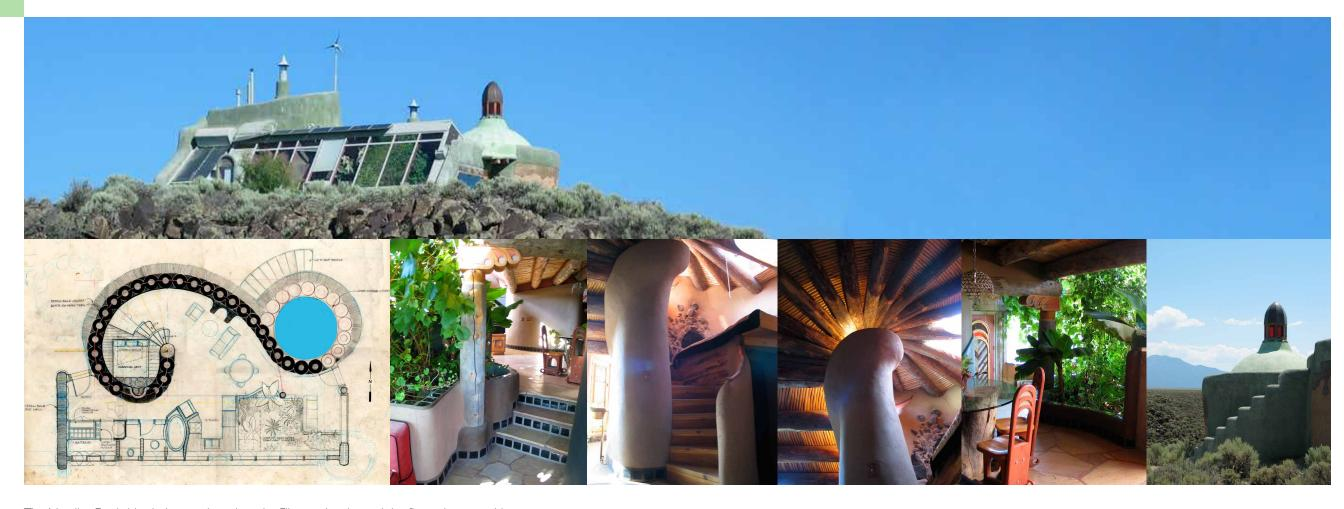
The Nautilus Earthship design was based on the Fibonacci series and the floor plan resembles a chambered Nautilus shell. It was built from the ground up on a lava rock site with rammed earth tires sheathed in straw bales. The spiral shaped floor plan wraps around a bedroom loft with a fireplace. The tire wall bends back in reverse to form a cistern for water storage.
